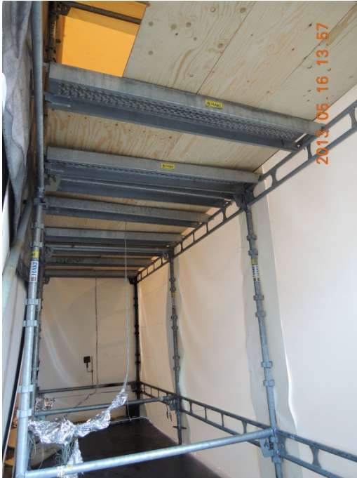
Figure 21 Inserted floor of plywood supported by a steel construction.
