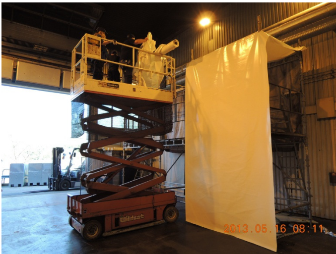
Figure 22 Fixing of vertical sheets.
