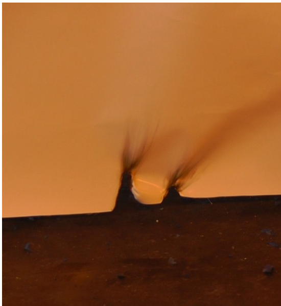
Figure 69 Fire damage after edge exposure from the outside (right: 15 s flame exposure; left: 30 s flame exposure).
