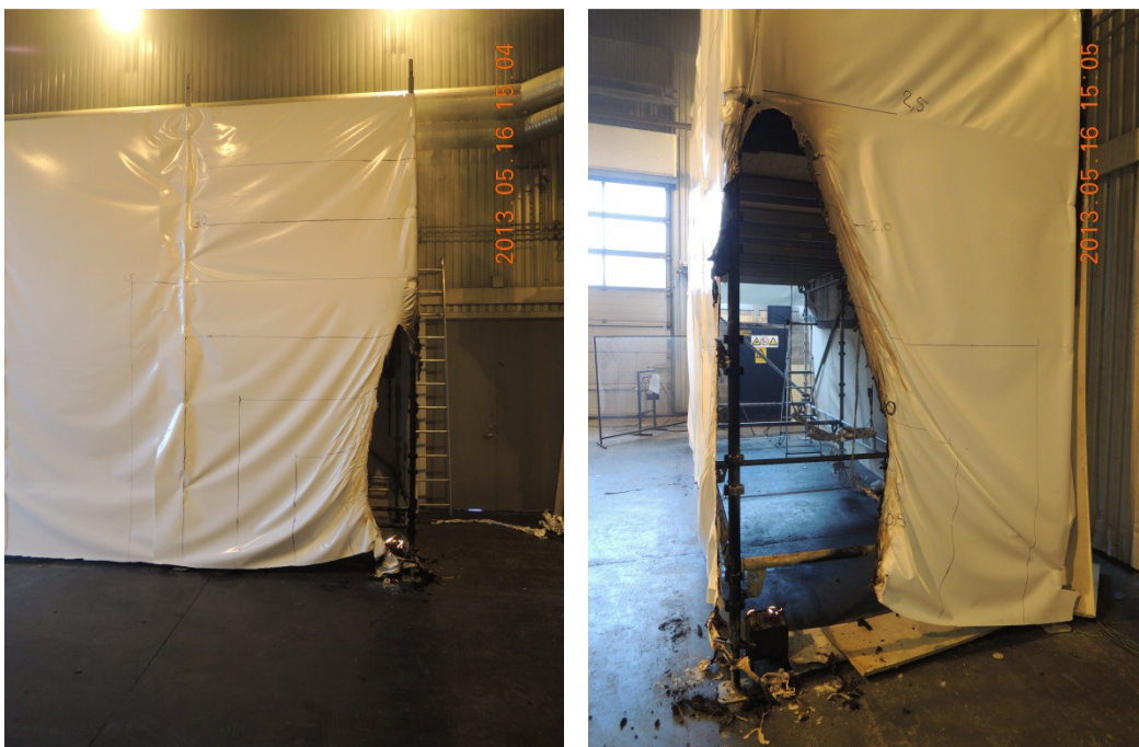
Figure 55 Fire damage of the material after the burner was turned off (left: front side | right: short side).
