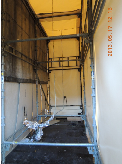
Figure 25 The thermocouple trees at position A (foreground) and position B (background) continued up to ceiling level.
