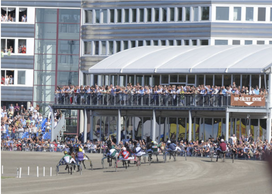
Figure 4 The two-floor textile building erected at Solvalla horse racing track.
